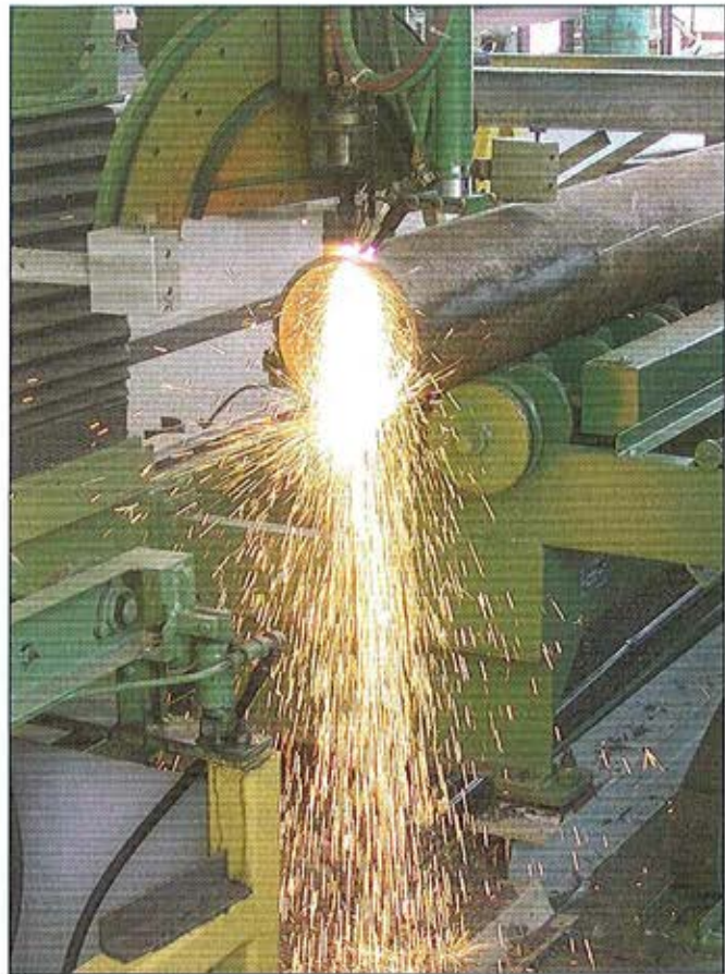
Fig. 5 — End of thin-wall diagonal member being thermally cut on CNC equipment. The length, end-for-end clocking, asymmetric "fish-mouths," and bevel angle are simultaneously cut.
